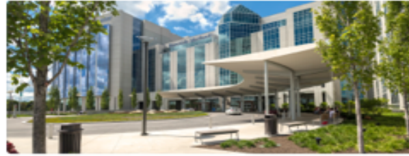
OhioHealth Riverside Methodist Hospital
